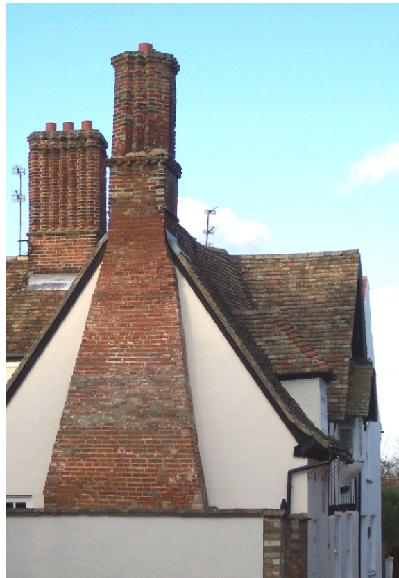
Chimneys at Plantagenet House
